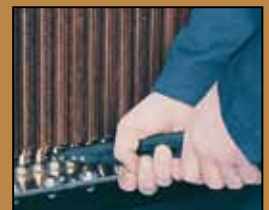
Tool seats tube into new lower seal.
